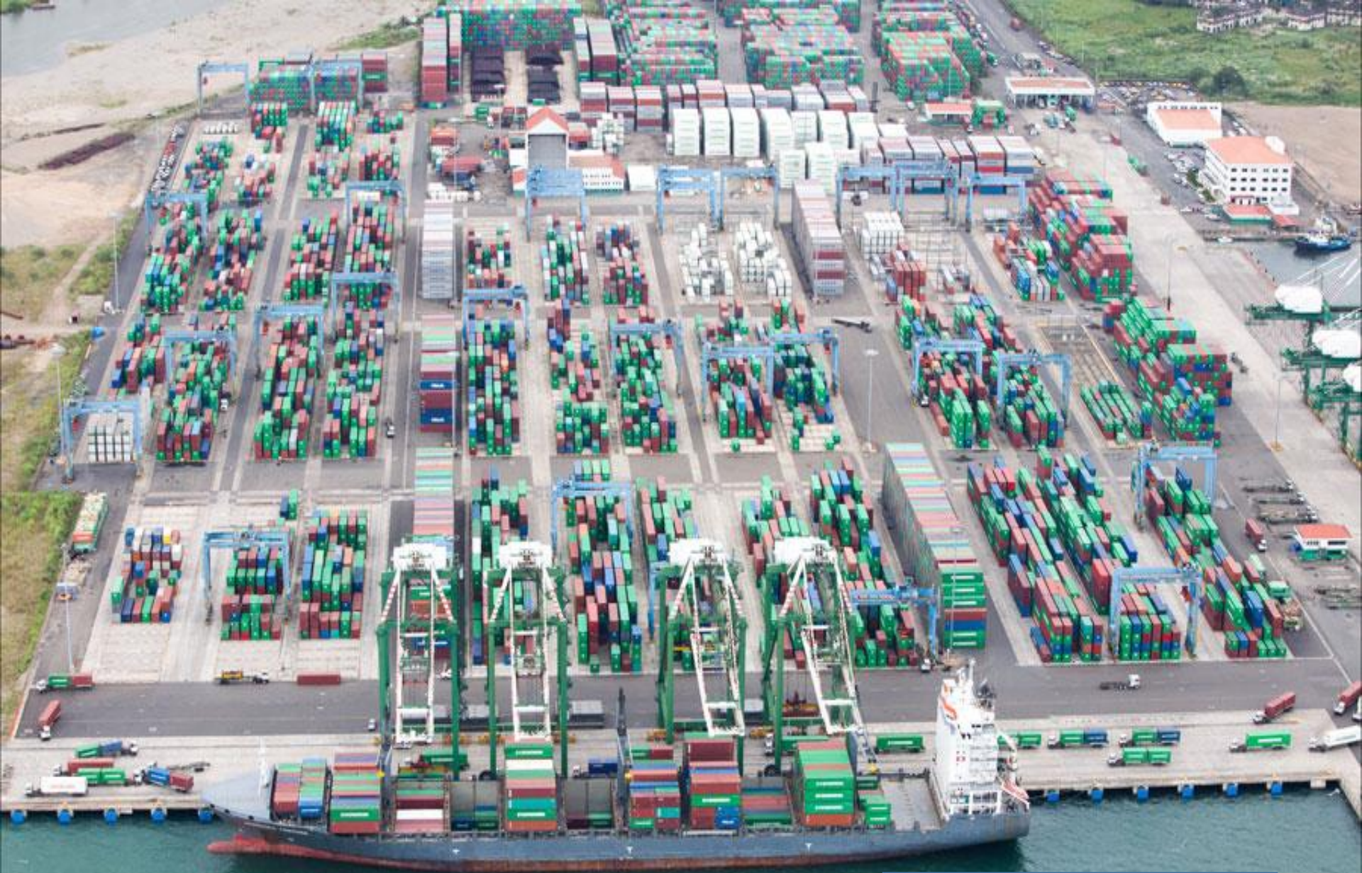
Colón Container Terminal
